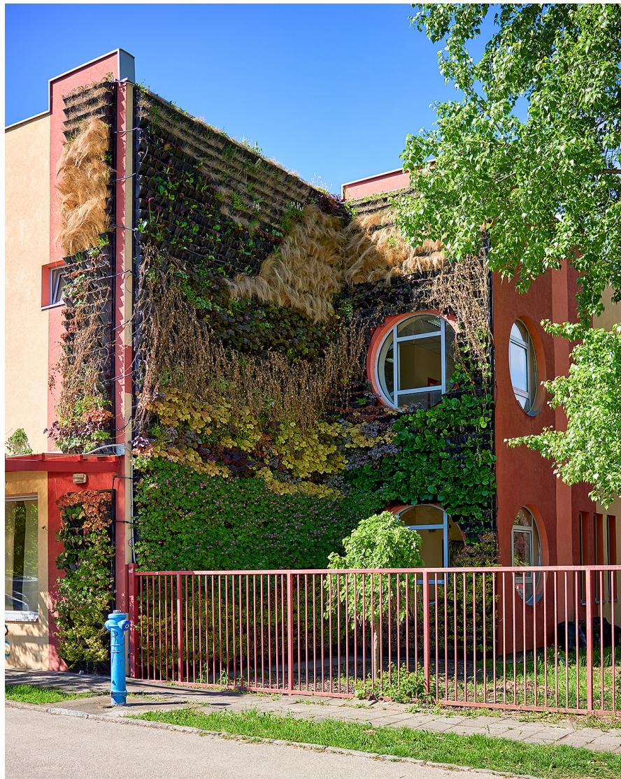
membrane, and the installation itself was mounted on the part of the street facade of the northeast orientation. For the purpose of the reconstruction of the green roof and the construction of the green wall, the replacement of part of the existing installations for water supply (irrigation) and sewerage (drainage) was designed and completed. Therefore, the installed green infrastructure will contribute to the additional energy efficiency of the facility (Appendix 8).
